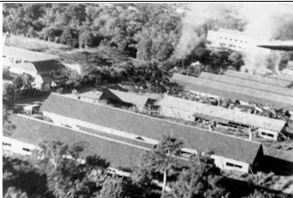
The Los Baños Camp was built in 1943 to house the overflow from Santo Tomas. It consisted of 20 barracks made from bamboo, nipa and sawali. When liberated, it held 2,146 civilian prisoners.
